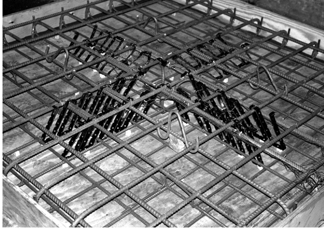
Fig. 6 Reinforcement in slab PSS-B
