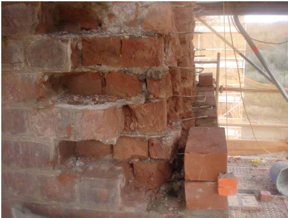
Figure 6. View of the pier rehabilitation works
