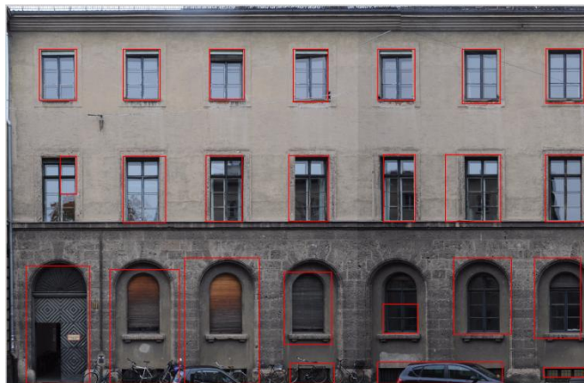
Figure 37: Oversize window patches due to niches
