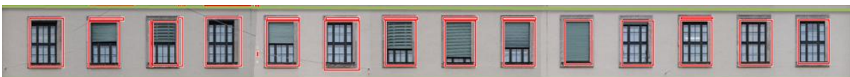
Figure 26: A chosen template in each block is cross-correlated to all areas enclosed by red bounding boxes in a respective block
