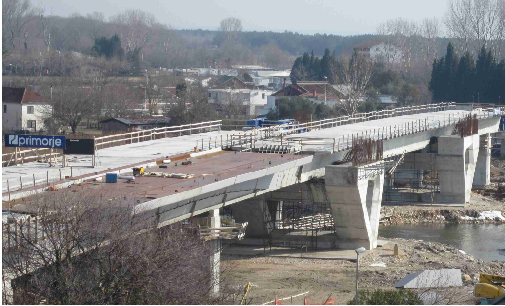
Slika 3.28: Most Port Milena med gradnjo. Figure 3.28: Bridge Port Milena under construction.
