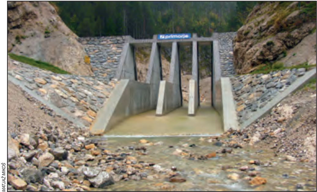
Figure 4: Downstream view of the 11.5 m high debris-flow breaker, made of reinforced concrete, finished in winter 2005, approximately 150 m upstream of the prefabricated bridge in Gorenji Log, at the upstream edge of the narrow in the Predelica Torrent, September 29, 2005. The debris flow breaker reduces the debris-flow kinetic energy and retains debris-flow coarse fractions thus changing debris-flow rheological characteristics downstream of the breaker.
