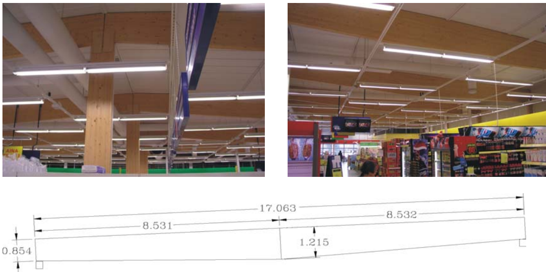
Figure 1. Kokemäki K-Market and the geometry of the tapered glulam beam analysed in this case study
