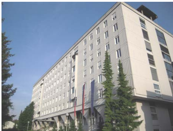
Slika 9.2: Obravnavana obstoječa armiranobetonska stavba Figure 9.2: The investigated multi-storey RC building
