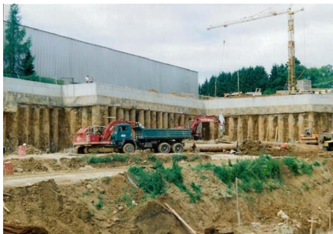
Slika 2.12: Sidrana pilotna stena – Krka – Notol 3
