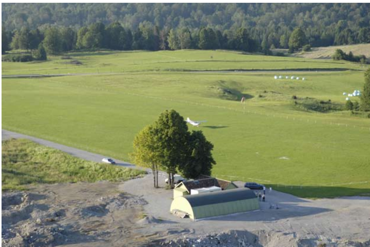
Slika 8: VPS Novi Lazi in obstoječa hangarja
