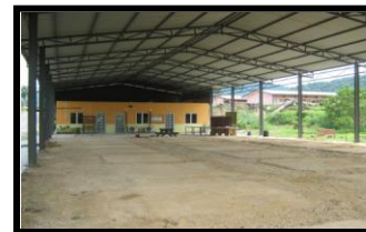
(c) At construction workshop in IKBN Dusun Tua
