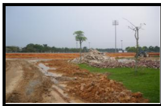
(a) At Construction site in Universiti Tun Hussein Onn Malaysia (UTHM)
