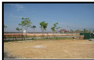
(b) At Construction site in Sri Gading
