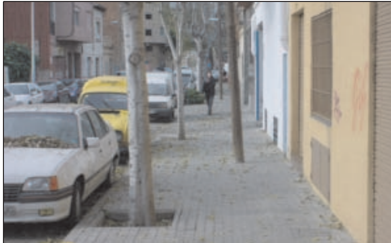
Picture 013 > Elements which are not aligned with and placed on the edge of the pavement can be the cause of an accident or disorientation of visually-impaired people
