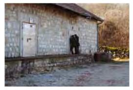
explosive and fire hazards. Most ammunition is stored on pallets, but some stocks are more than 2 metres high due to a lack of capacity. Lightning protection is in place at all buildings. The doors are made of wood, covered with an aluminium cover plate and are not up to NATO standard.
