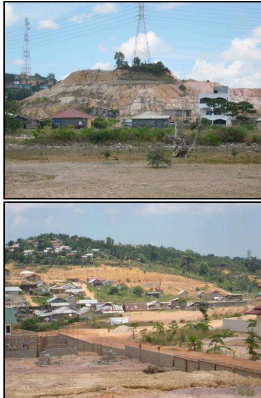
Figure 10: The cutting of the hills in order to get the reclamation material.
