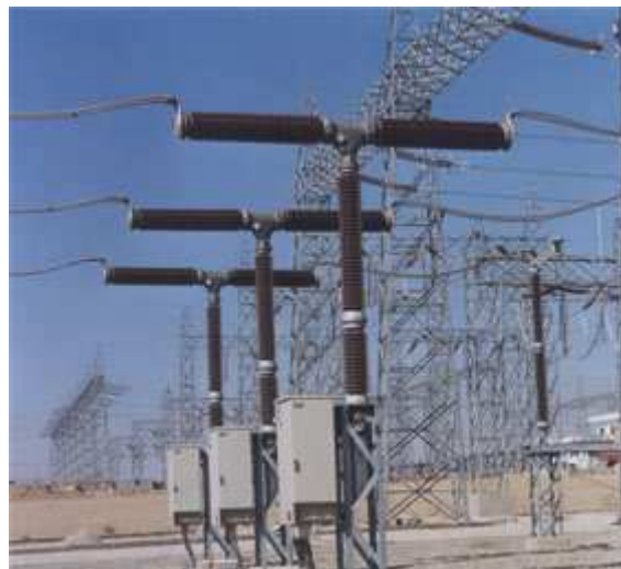
Figure 2.4: Live tank circuit-breaker (Source: ABB AG, Switzerland)
