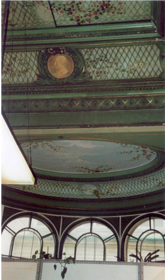
Abb. 125: Palais Corbelli-Schoeller, 1. Stock, Wintergarten. Erker.
