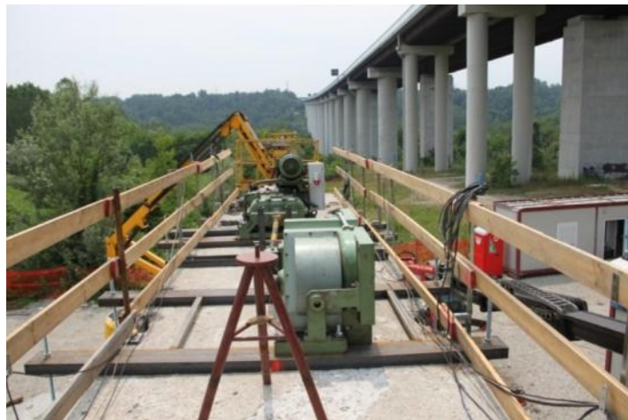
Figure 29 Beam B05: the vibrodyne placed on the slab
