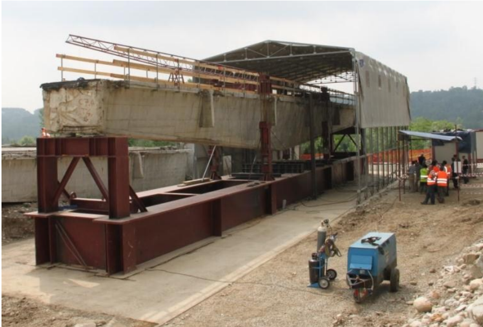
Figure 4 A beam placed on the test bench
