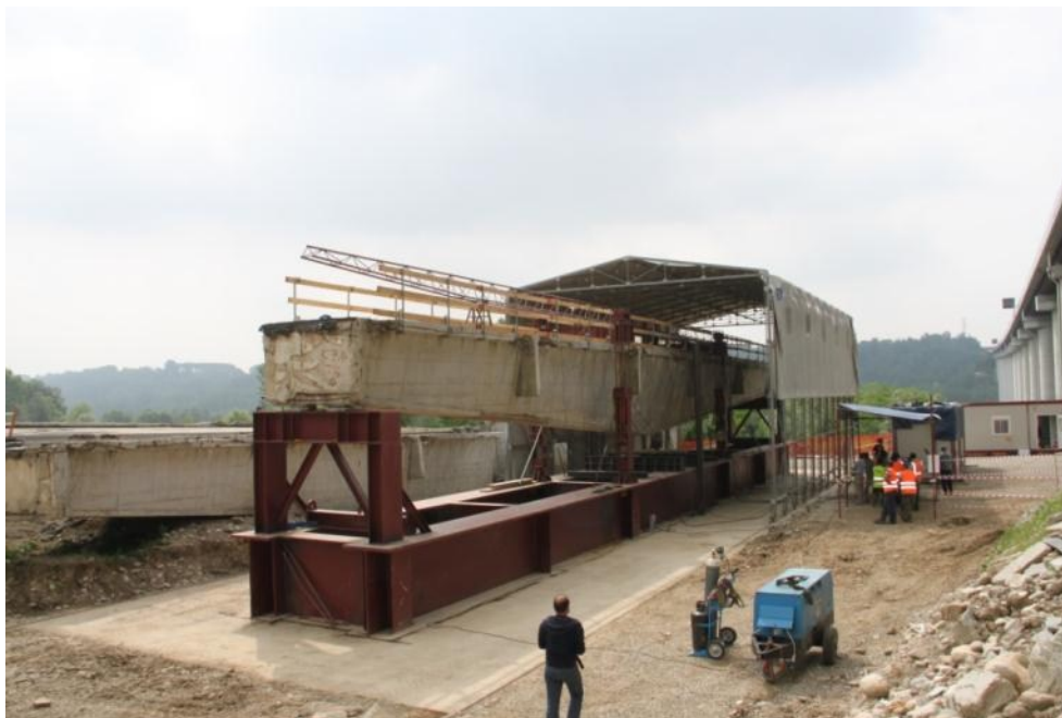
Figure 16 Beam B03 placed on the test bench
