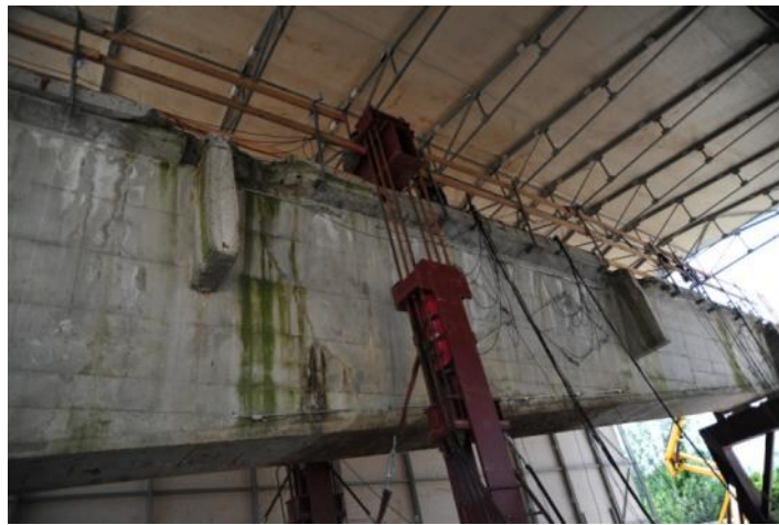
Figure 28 Beam B05: view of the beam on the bench test
