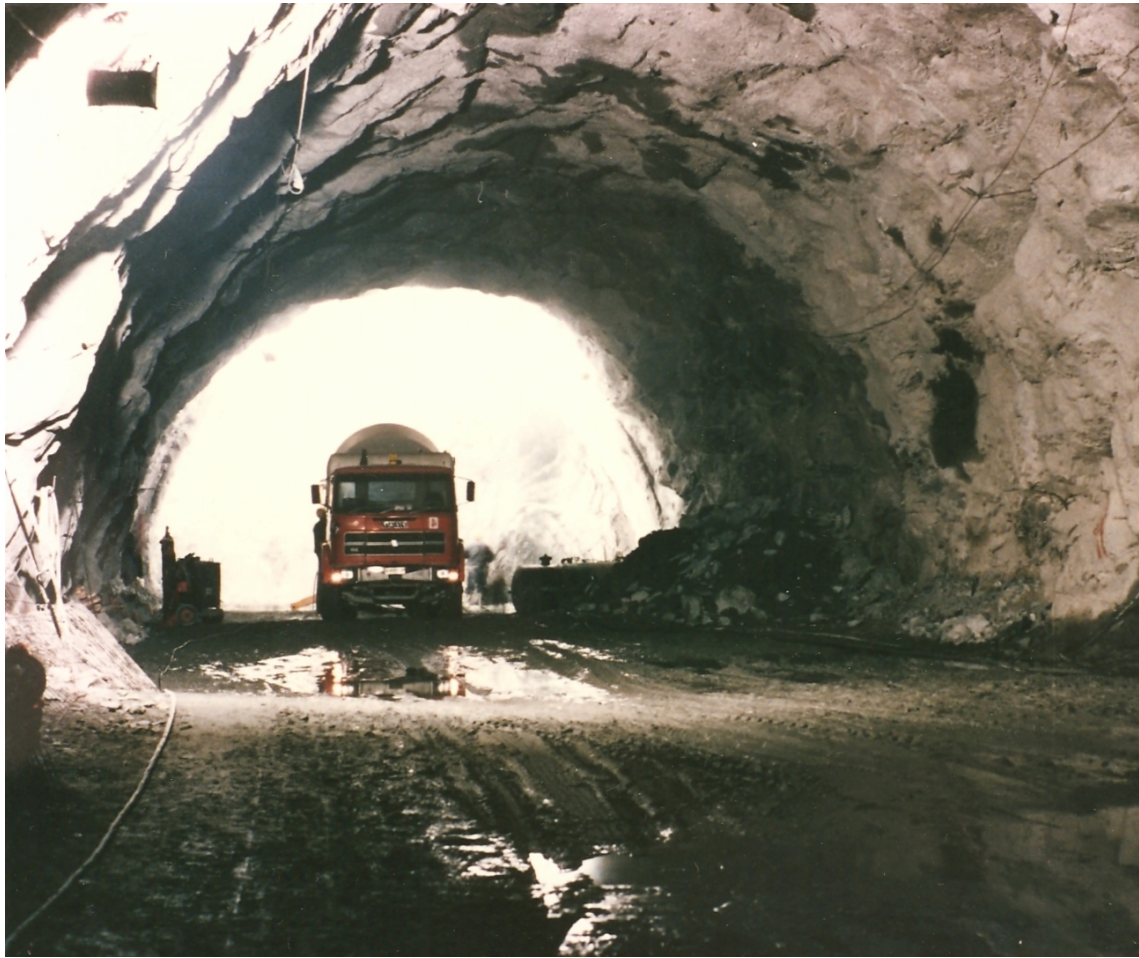
Fig. 4. Example of usual irregularity of the boundary for a road tunnel excavated by drill and blast in black calcareous shists (courtesy Prof. S. Pelizza).
