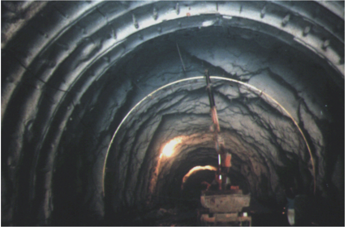
Fig. 3. Photograph of large overbreaks induced by joints discontinuities around a road tunnel. The steel rib indicates the theoretical tunnel boundary (courtesy Prof. S. Pelizza).
