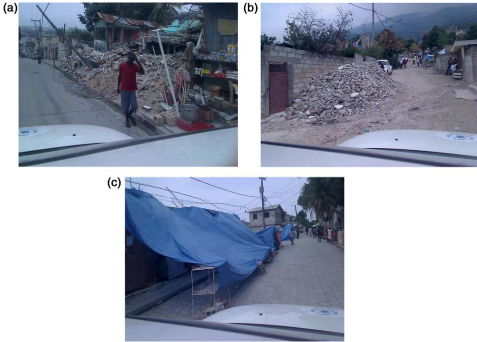
Figure 7. Examples of LCMMS georeferenced frames acquired during the survey. (a) Collapsed building, (b) Restricted road, (c) Temporary shelter.
