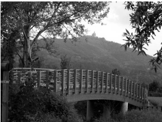
Figure 5. A new pedestrian bridge.
