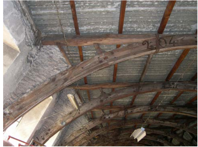
Figure 8 – The former Gallo wool mill, Sagliano Micca (Biella). Detail of the assembly system of the boards. (photo Mattone).
