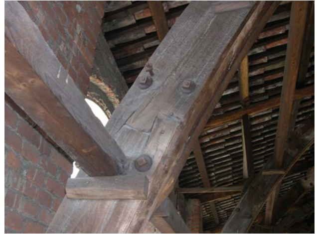
Figure 5 – The former Trombetta wool mill, Biella. Detail of the arches. (photo Mattone).
