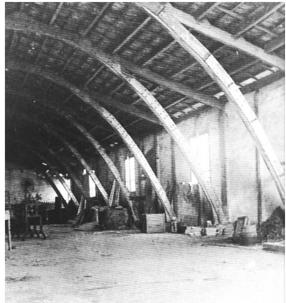
Figure 10 – The Pavilion of the Societat Obrera Mataronense, Matarò, Spain. The wooden arch structure.
