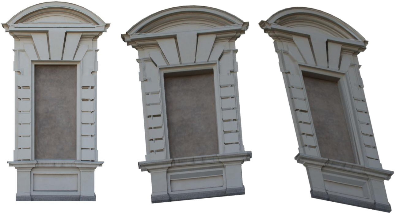
Figure 8. Photo-realistic views of one of the surveyed windows
