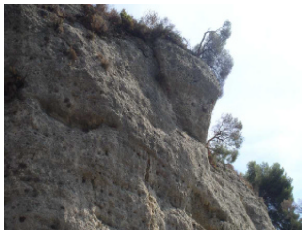
Figure 5. Detail of the unstable element (ref.3 in fig.4)
