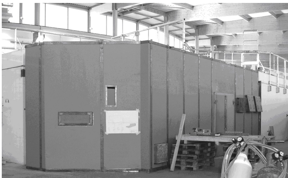
Figure 2: Picture of the optics hatch at the end of its construction
