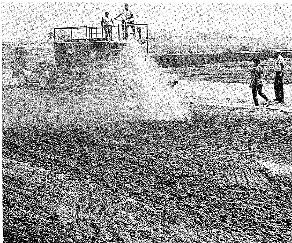
Figure 6. Roadside being seeded with hydromulcher.
