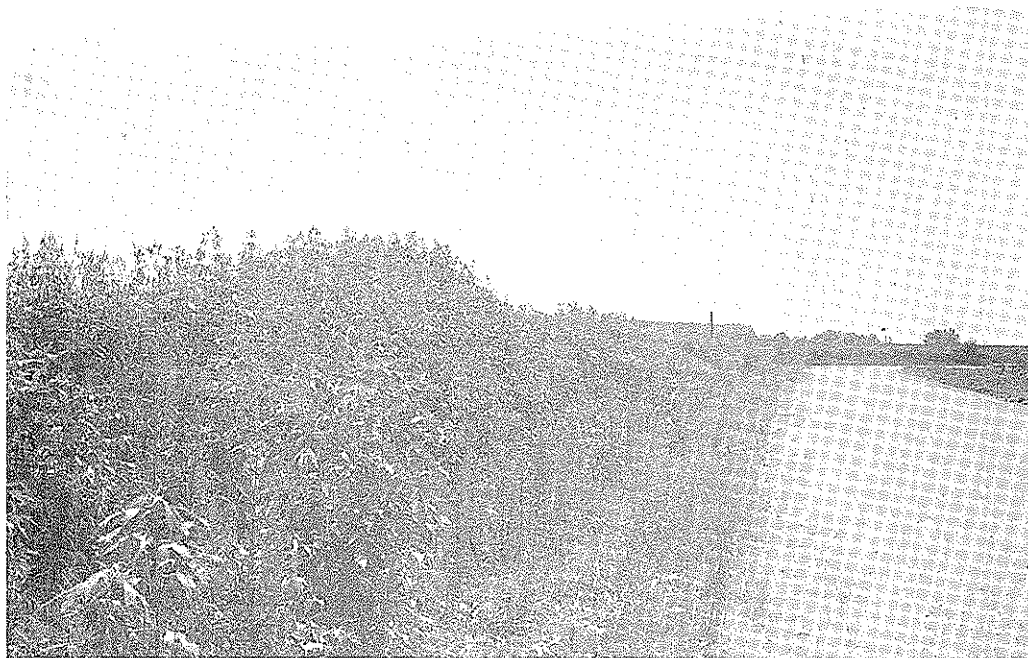
Figure 17. Weedy roadside resulting from ditch cleaning spoils being piled on the backslope.
