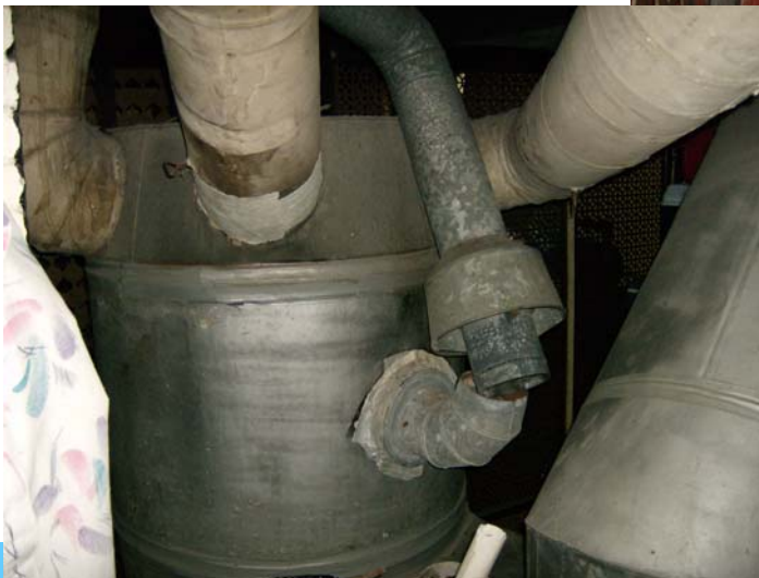
This is what happens when there is gas build-up; the door was blown off and so was the venting. The 80-year old couple living in this home were very lucky.
