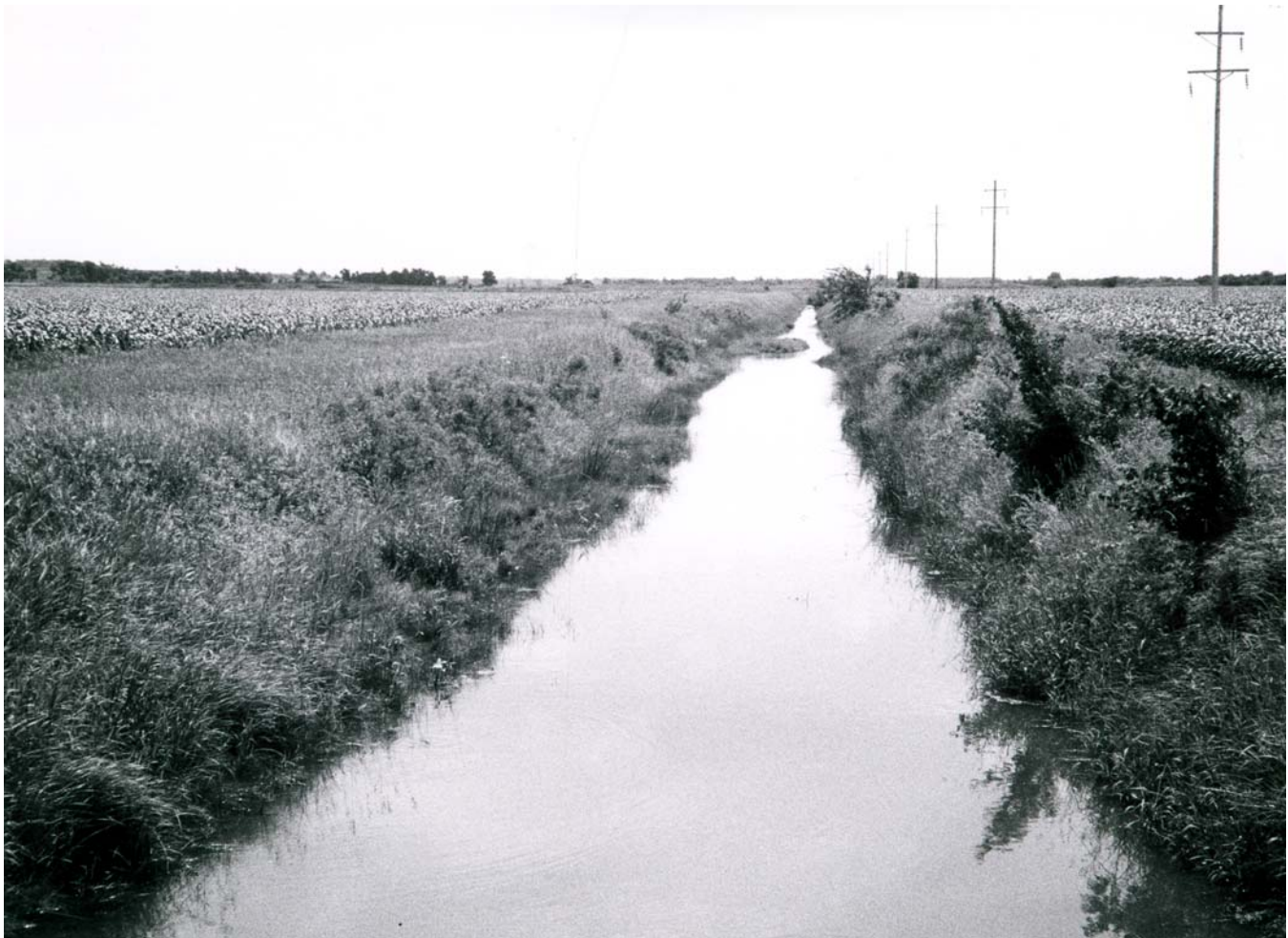
Figure 3.—Manmade drainage ditches help to lower the water table and control flooding on the nearly level flood plains in areas of the Colo-Zook-Spillville association.
