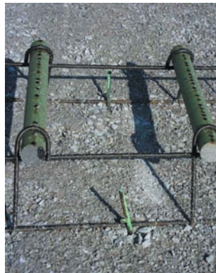
Staking dowel baskets (paver traveling ↓)
