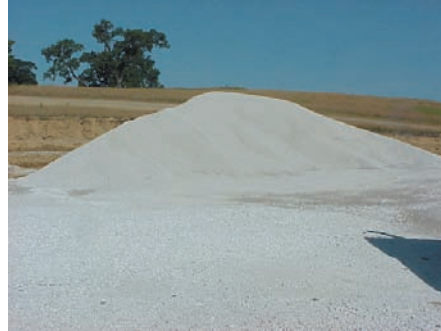
Well-built and well-maintained aggregate stockpile
