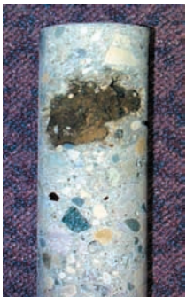
Mudball resulting from stockpile contamination
