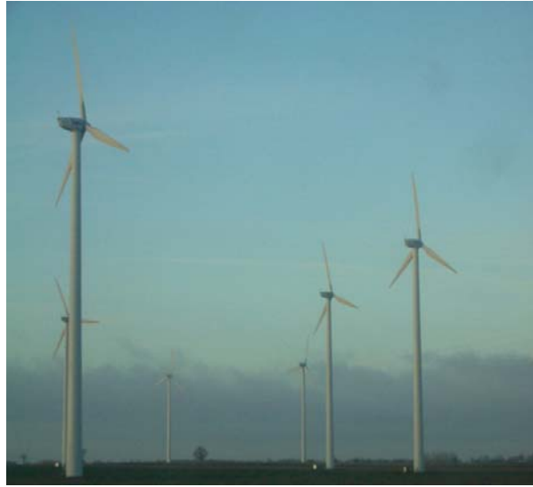
Figure 2.4: Wind Turbine Generators (Photo taken at Mecklenburg, Germany, 2006)
