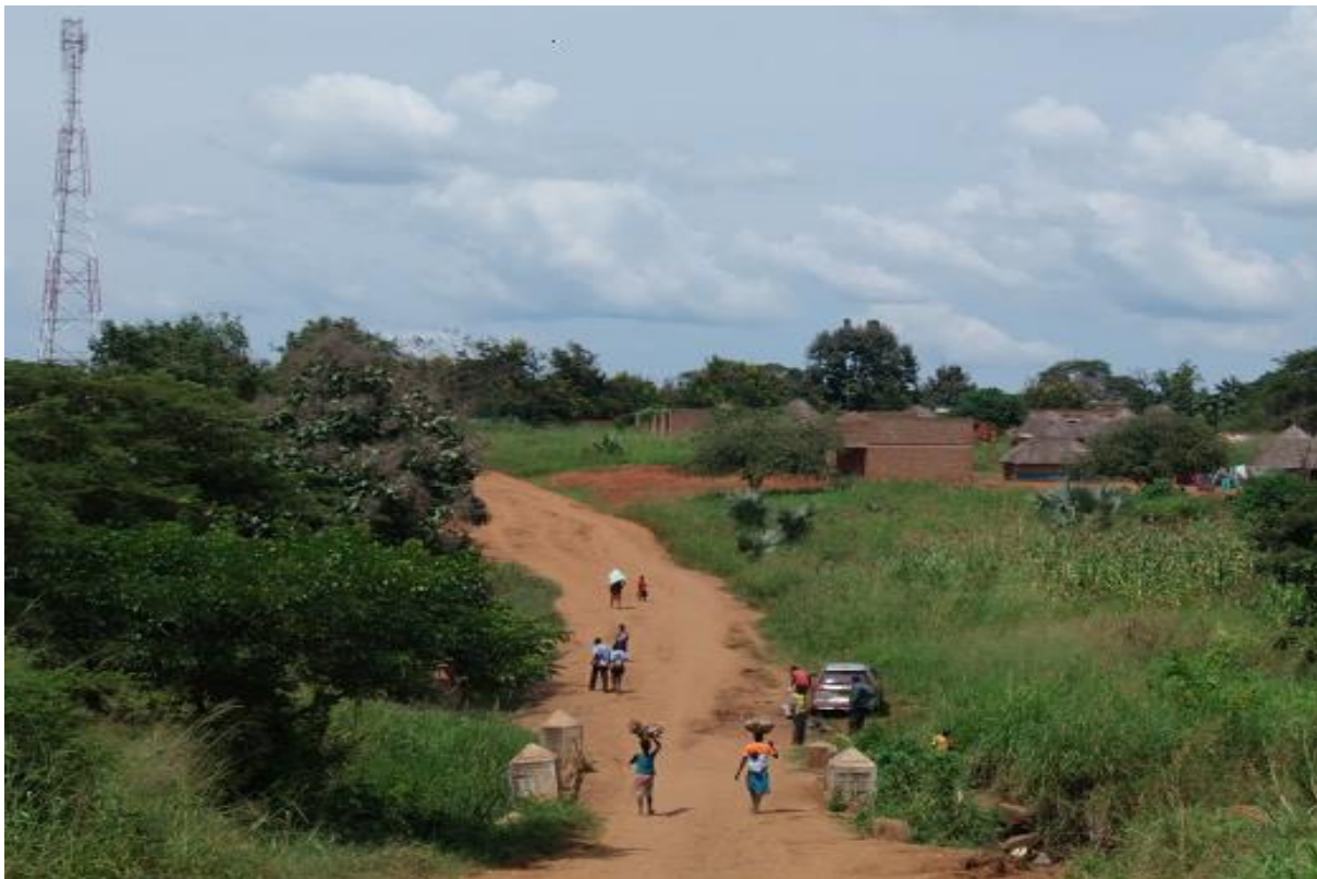
Fig 6: The bridge across the River Atebi. A new bridge has since been built and then destroyed by flooding. Note the MTN Communications tower in background, November 2013
