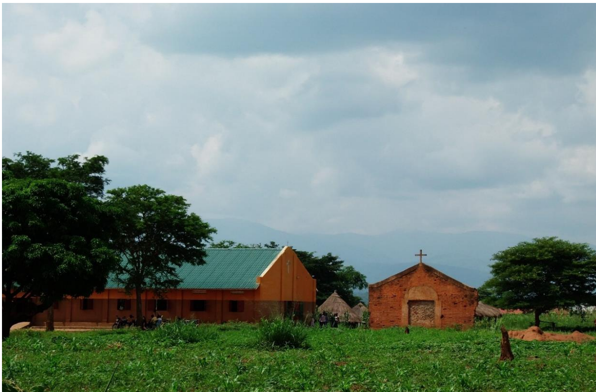
Fig. 27: St Andrews, AIC Caigon. The old church (right) was destroyed in Anyanya II, August 2014
