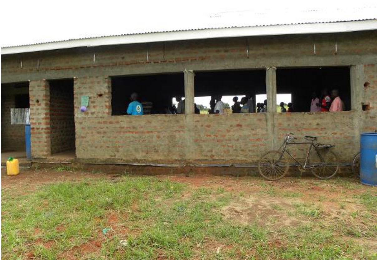
Fig. 31: The just-completed GTM church building, during the GTM Bible workshop, October 2014
