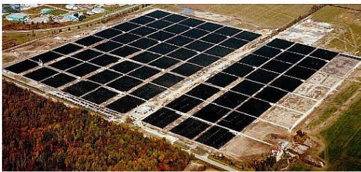
Fig 5.2 Sarnia Photovoltaic Power Plant http://www.pv-tech.org/news/a/enbridge_ups_first_solar_built_20mw_sarnia_project_to_80mw_by_end_of_2010/
