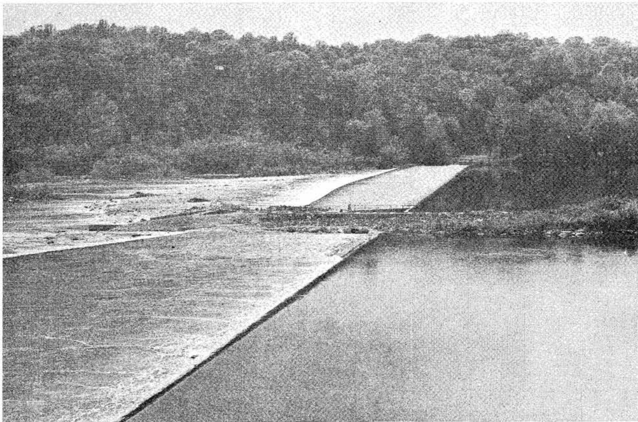
Figure 21.--Little Falls Dam, Potomac River, Md. Fishway between dams was completed in 1959.
