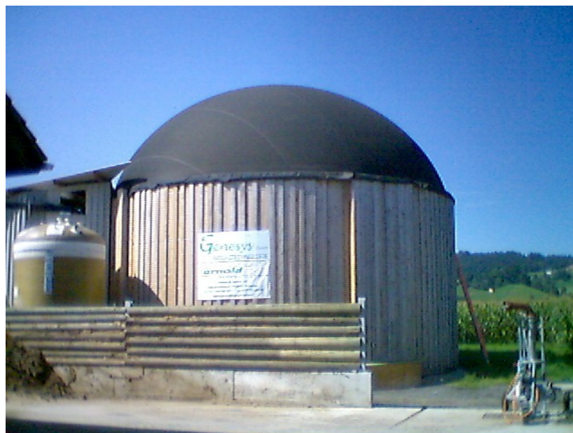
Example: Biogas plant at Altshofen (LU, 2006)
