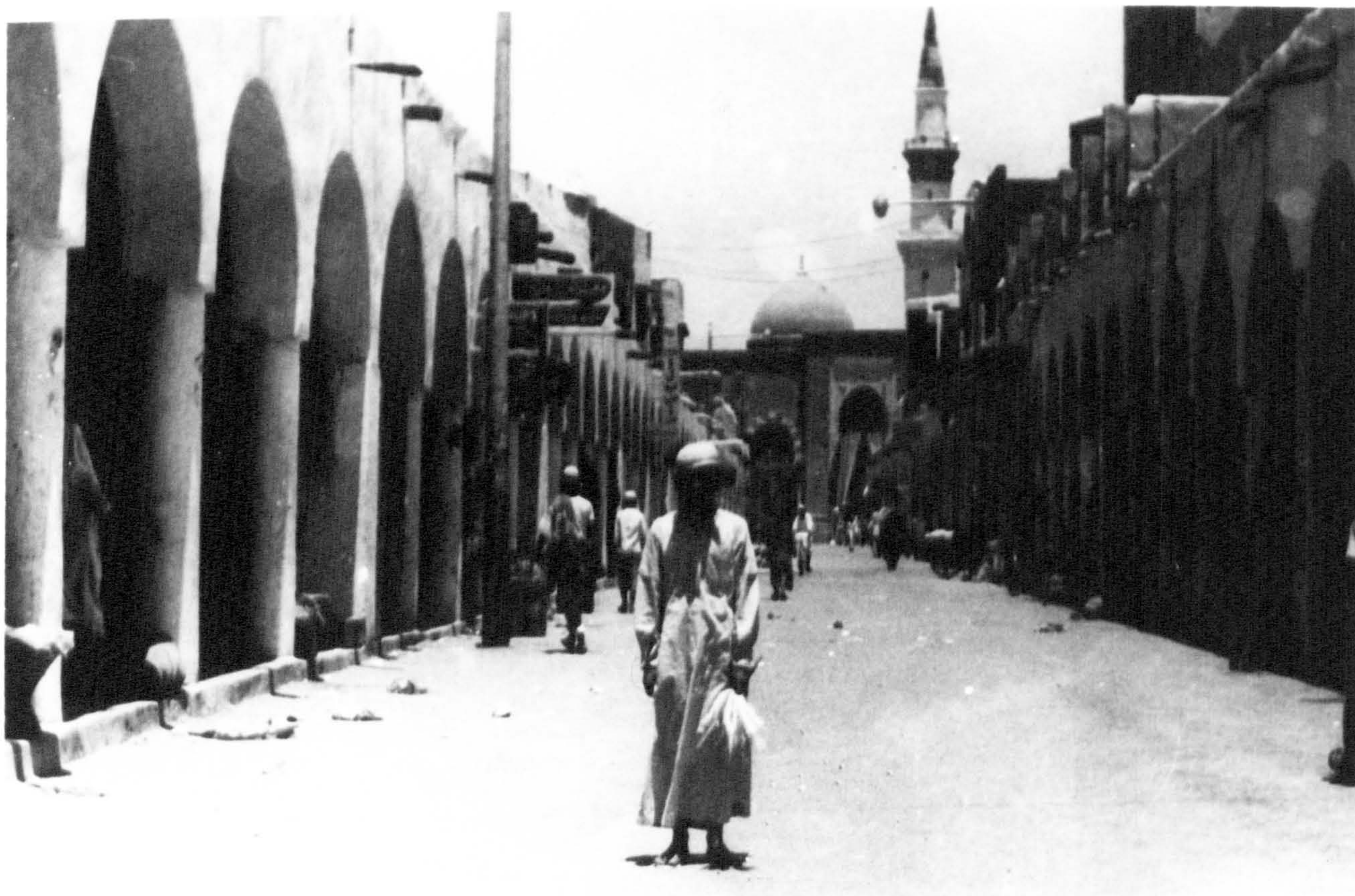
Plate 4.2 Arched sides of Al-Ainyyah street ( compare with Plate 4.1 where the arched sides have been demolished in the late 1960's initially to widen the street. Later in 1976 the whole street was demolished to make way for the enlargement of Al-Haram).
