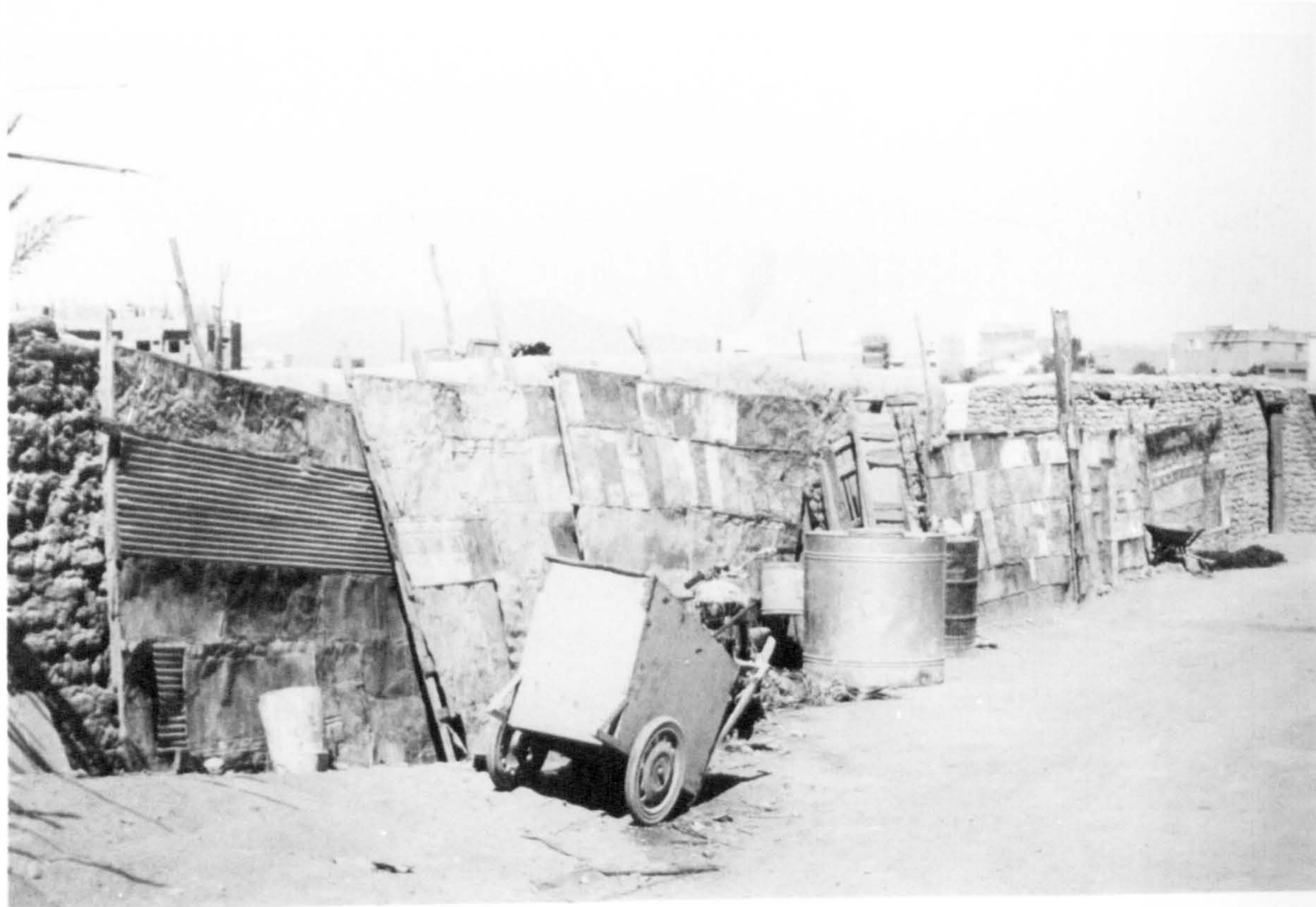
Plate 9.1 Tin sheets and sun dried bricks used for hut construction in the Eastern Harrah of Medina.
