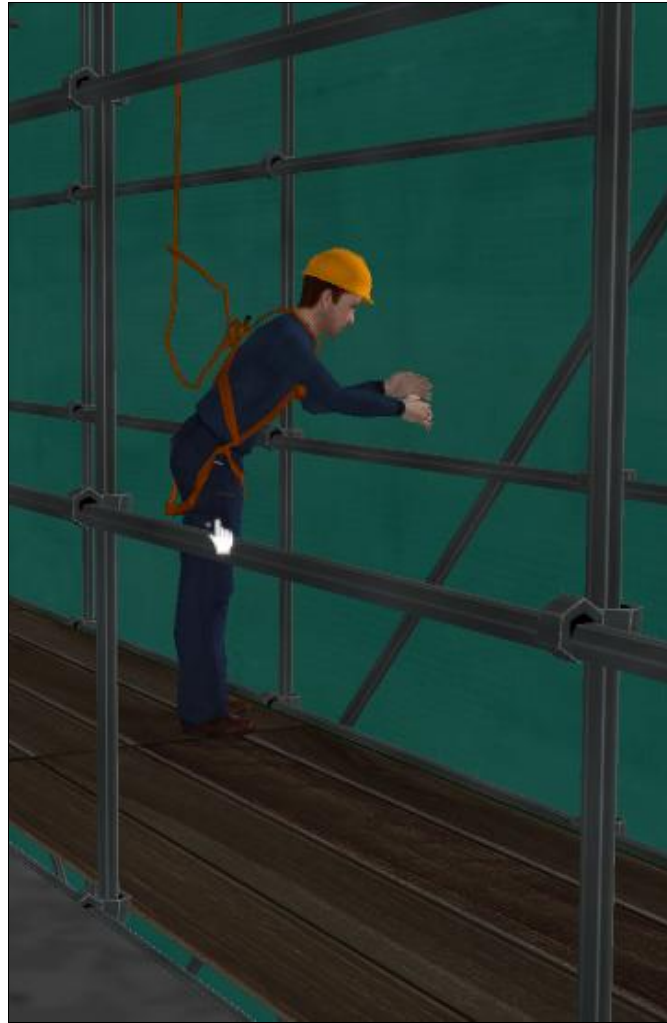
Figure 7. Working at height without a safety belt
