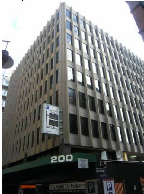
Figure 6.2 Exterior of CH1 building
