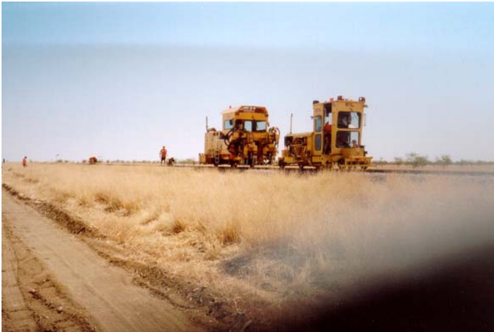
Figure 2.21 Straightening, Tamping and grinding
