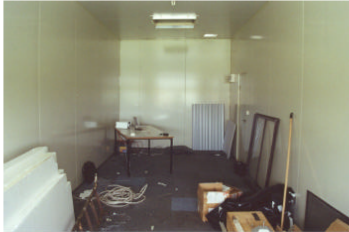
Figure 5.21 - Uniform Illumination of Test Building with Vertical Micro-Light Guiding Shade Panels under Clear Sky
