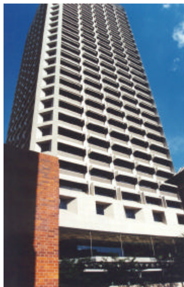
Figure 2.3 - Tilted Canopy Shades Drastically Reduce Internal Natural Illumination
