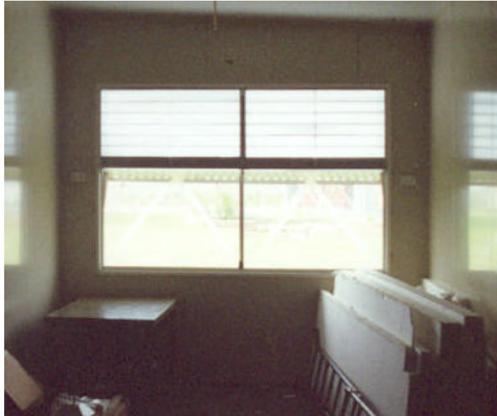
Figure 5.27 - Contrasting Dark Band at Bottom of Vertical Micro-Light Guiding Shade Panels
