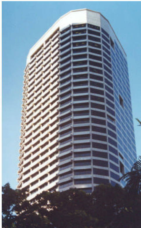
Figure 1.1 - Heavily Shaded Sub-tropical Office Building
