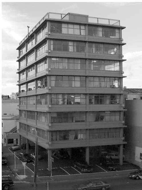
Figure 1. Existing Pre-1976 Building
