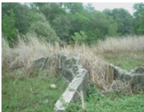
An abandoned fish pond reverts to mangroves
