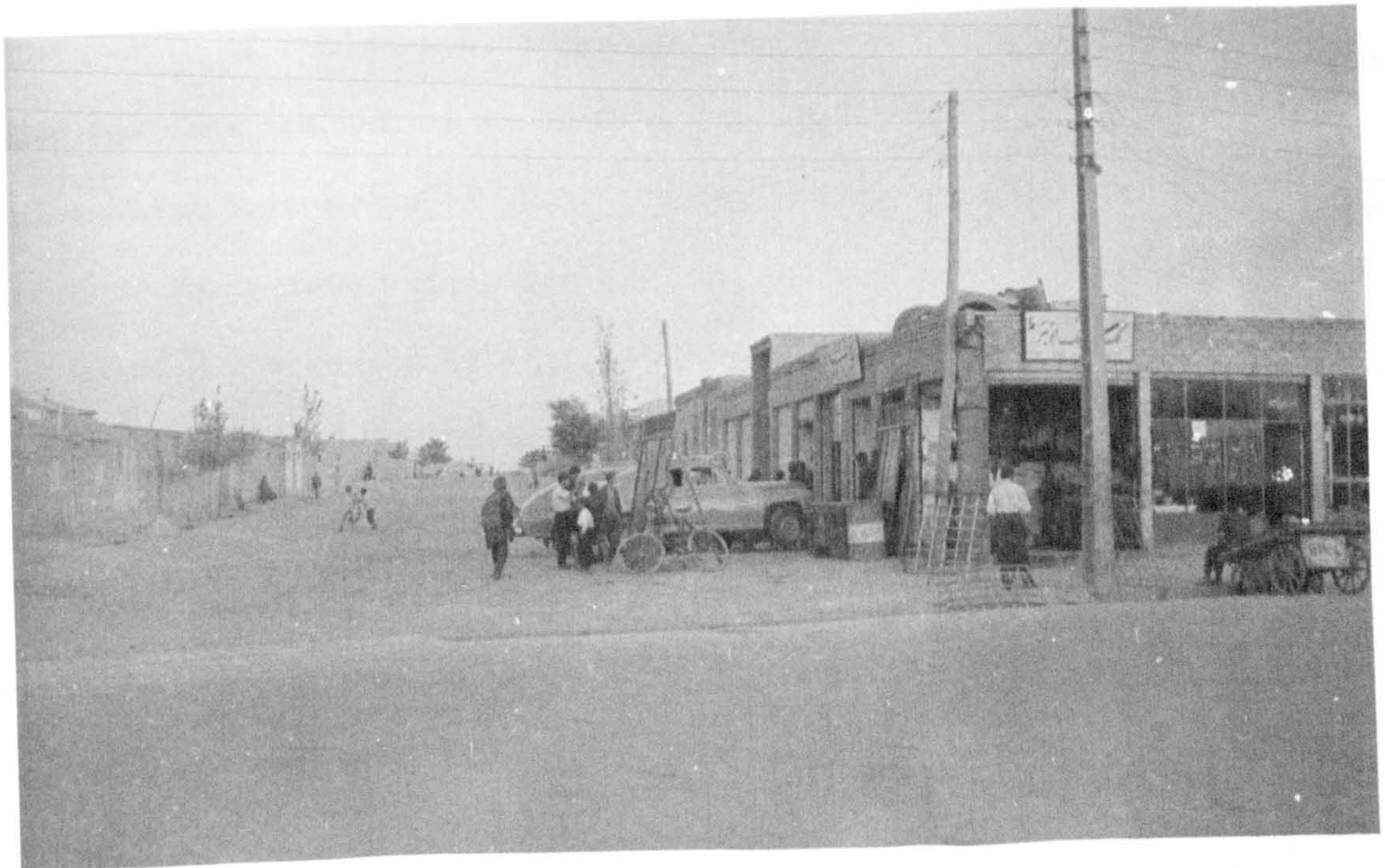
Plate 24. The new khiaban running south off Pain Khiaban.
