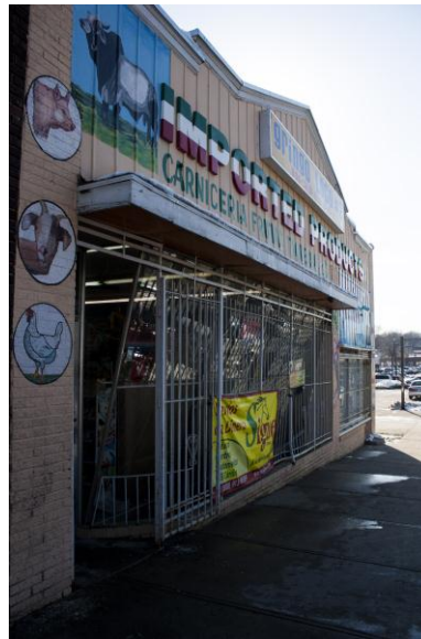
Figure 3.18 Barred Windows photo by J. Nelson.
