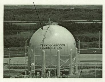
The LC-39 Pad B 900,000 gal. LH2 Dewar exhibits a boil-off loss rate over twice that of an identical Dewar on Pad A. This has been know since the tank was built (1964) and has resulted in millions of dollars of loses.
