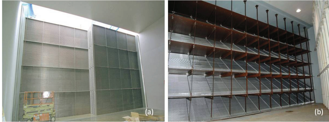
Figure 2: (a)previous flat-panel heat exchanger, (b)current chevron-design heat exchanger
