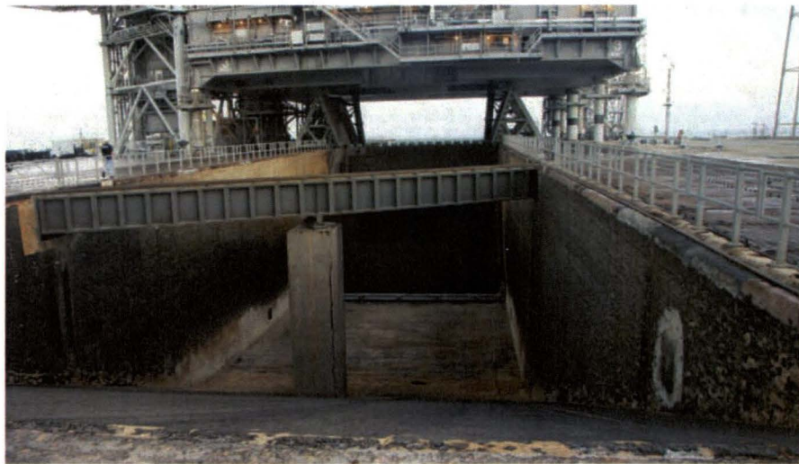
Figure 5. SSME Flame Trench
