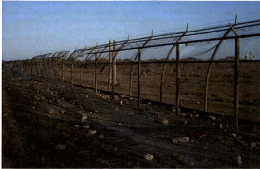
Figure 11. Refractory Concrete Bricks Around Fences
