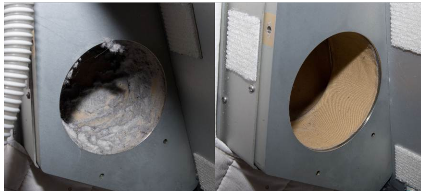
Figure 3. Starboard CQ intake duct (pre and post cleaning).
