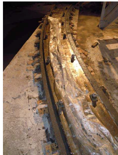
Figure 2. a) Continuous metal plate installation and b) grouting phase
