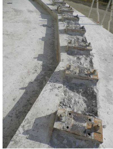
b) Grout removal, metal plates visible
