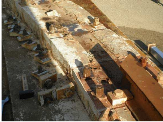
Figure 1. a) Rail track removal
