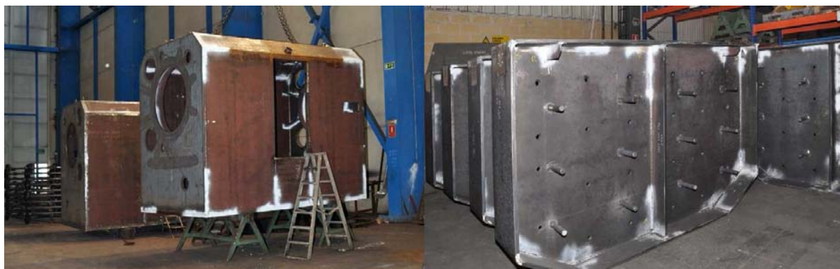
Figure 3. RAEGE telescopes under construction in Spain. Left: receiver cabins. Right: antenna counterweights.
