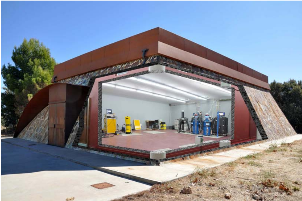
Figure 2. The A10 absolute and GWR superconducting gravimeters installed in a dedicated building in Yebes. (Figure courtesy of Carlos Albo Castaño, IGN).
