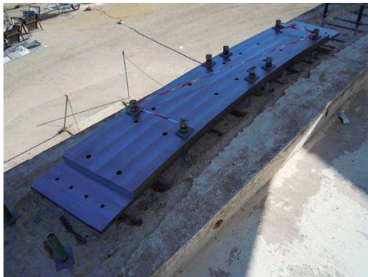
Figure 2. a) Continuous metal plate installation and b) grouting phase
