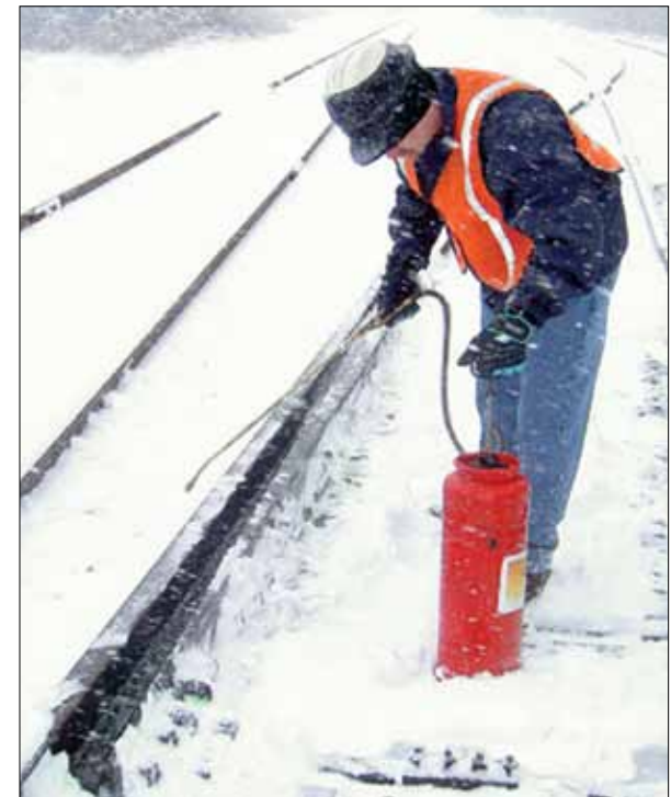
Railroads use Ice Free Switch, incorporating NASA technology, to stop water from becoming ice on train track switches. This helps to maintain train service during winter weather events.
