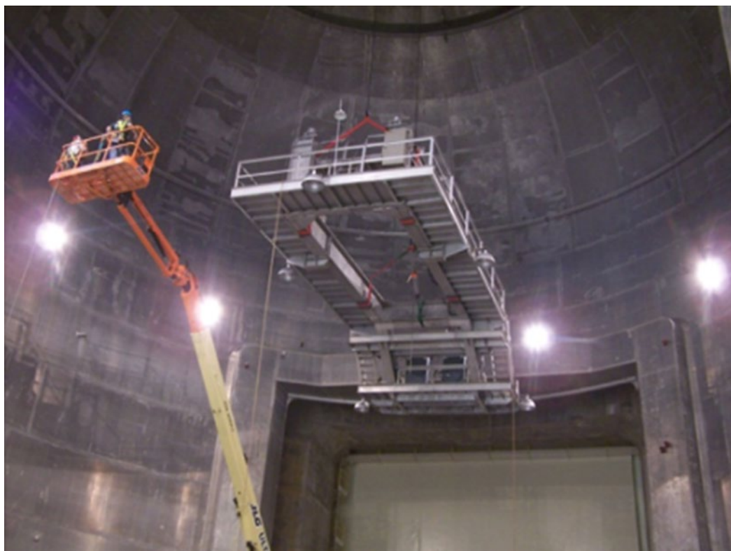
Figure 3.—Lowering of the polar crane bridge.
