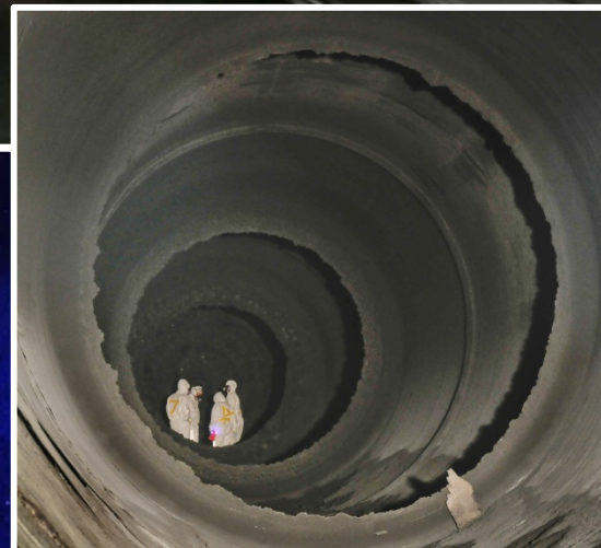
Post-test inspection of DM-1 insulator
