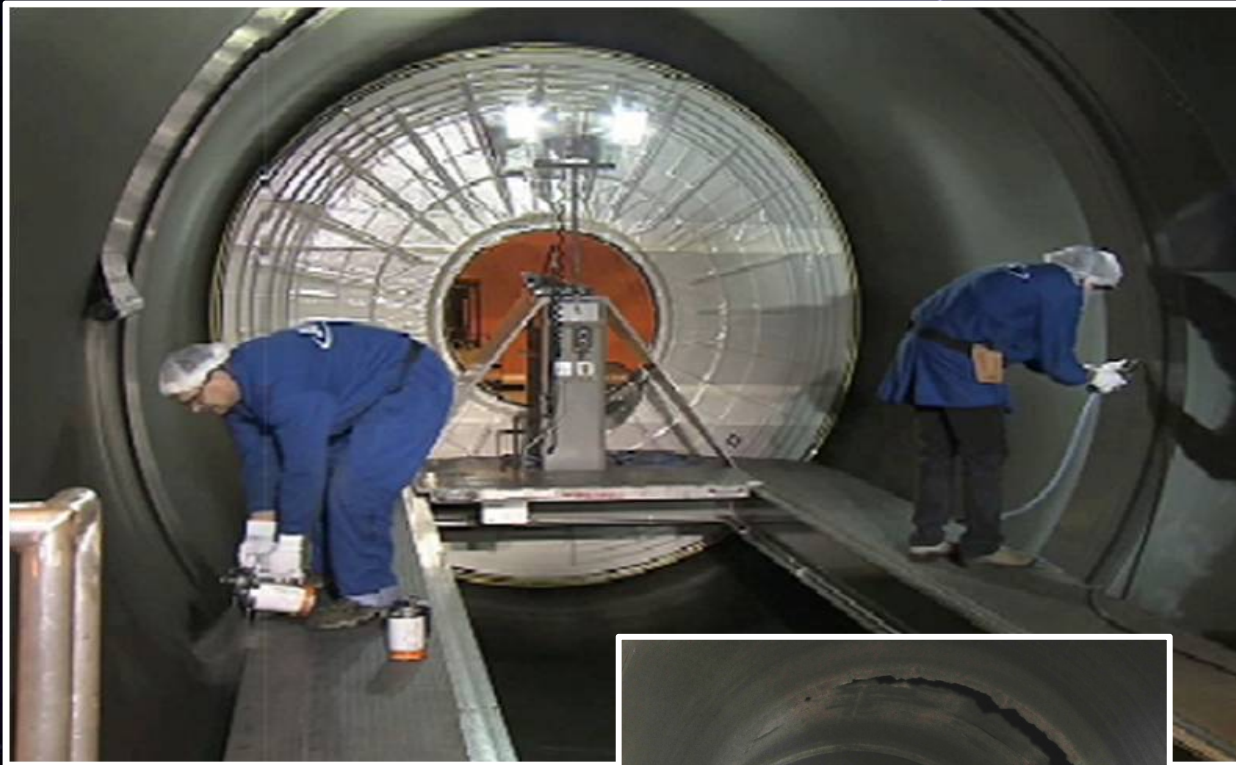
Layup process of PBI - NBR insulator
