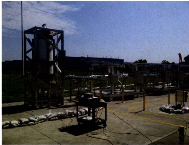
Figure 3-4: GODU LOX Insulated AFRL composite tank and chill down line.
